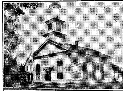
THE OLD CHURCH BUILDING Medina, Ohio
